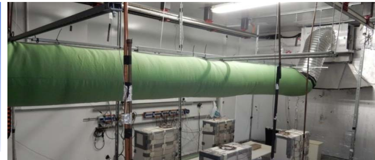
Air distribution via whole fabric duct at medium level.
